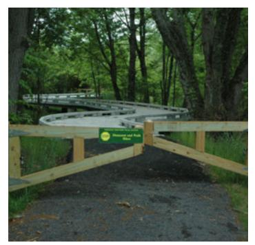
The pedestrian bridge was constructed of unpainted weathering steel with hardwood decking. The boardwalks were created from prefabricated concrete that was assembled in place, allowing for fast construction and minimized removal of mature trees.
